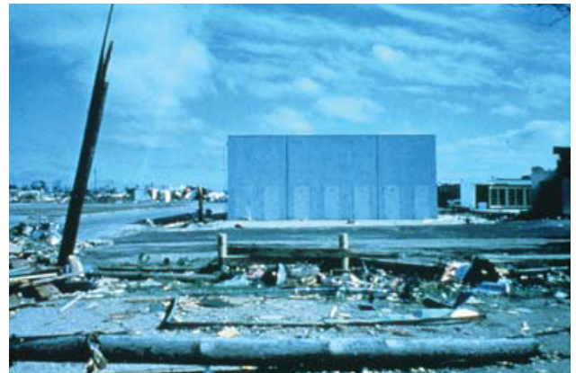
"Tilt-Up" commercial building standing fully intact after a destructive tornado. (USA)
